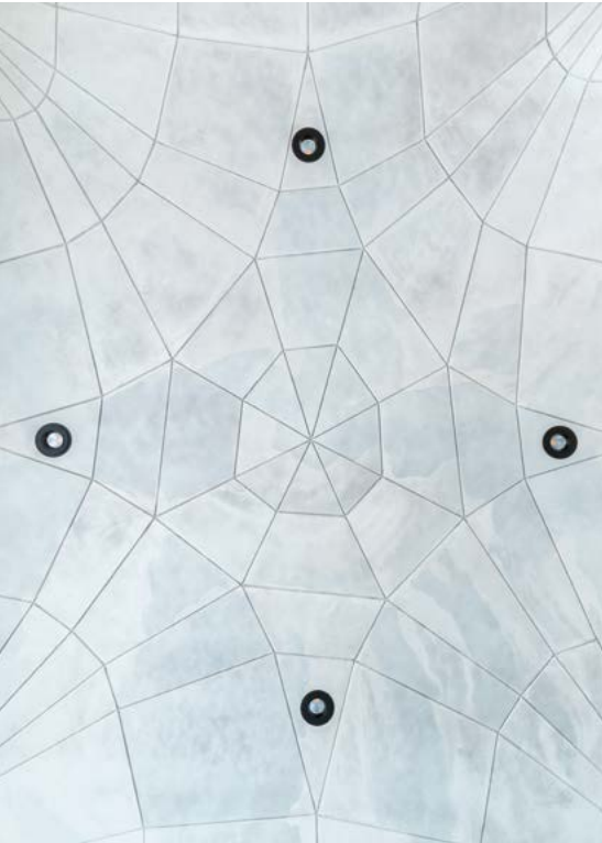
The HiLo unit of the NEST research and innovation building in Switzerland is built with ECOPact green concrete in the lightweight floor system with 33% lower CO 2
