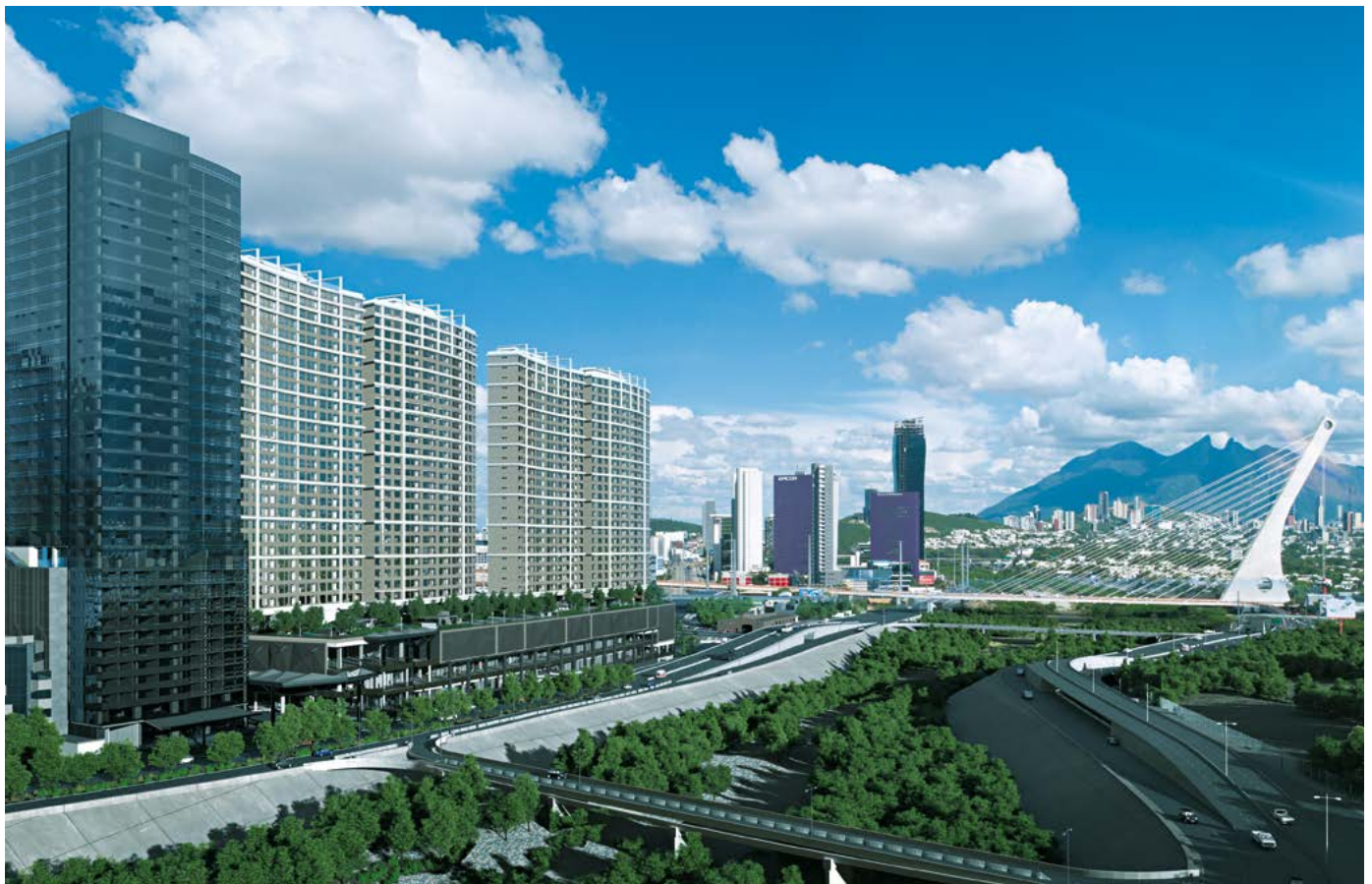
Torre Avalon, Mexico, is built with iConcrete digital solution and ECOPact green concrete with 30% lower CO 2
