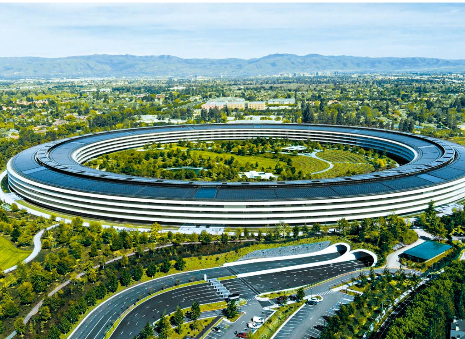
Apple Park, Cupertino, US, is built with Firestone EPDM enabling its solar roof
