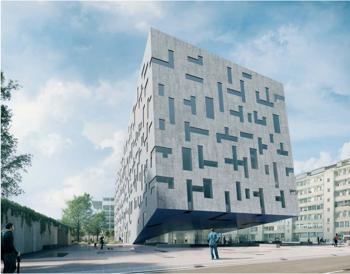
New CAP Group Headquarters, Milan, is built with ECOPact green concrete with 35% lower CO 2 to achieve LEED Gold certification
