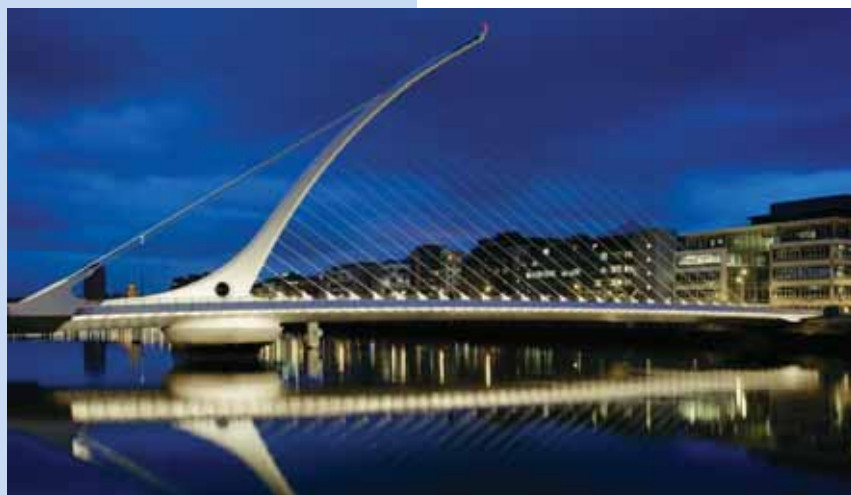
Samuel Beckett Bridge (Wikipedia)
